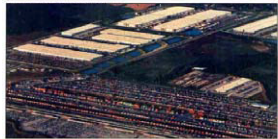
Chicago's industrial real estate profile has been bolstered by projects like the redevelopment of the former Inlet Arsenal into CenterPoint Intermodal Center in Elwood, IL.
